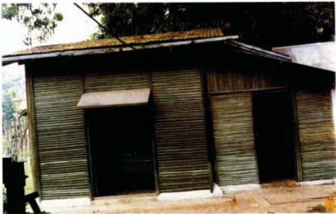
FIGURE 12 (b). Low cost hut made out of CCA treated bamboos (erected 1955)
