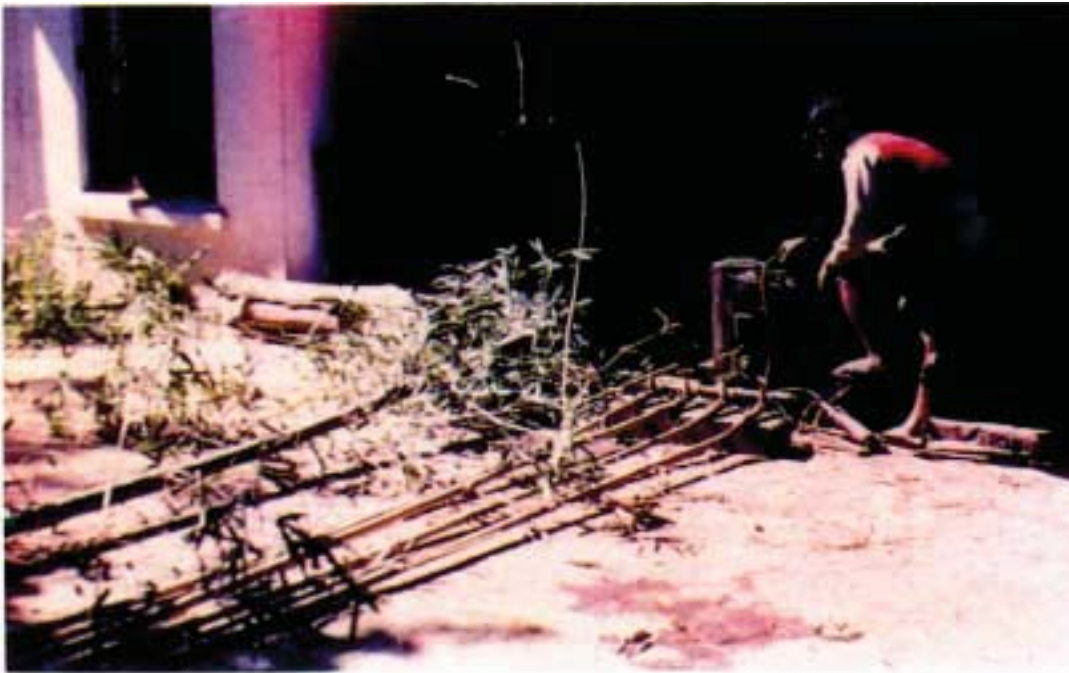
FIGURE 6. Boucherie treatment of green bamboo using foot pump for creating pressure.
