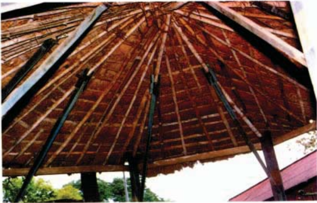
FIGURE 12 (a). Round and split bamboos used under thatch roof (erected 1955)
