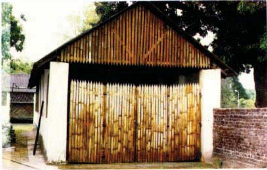
FIGURE 8. Use of treated bamboo (erected 1989)
