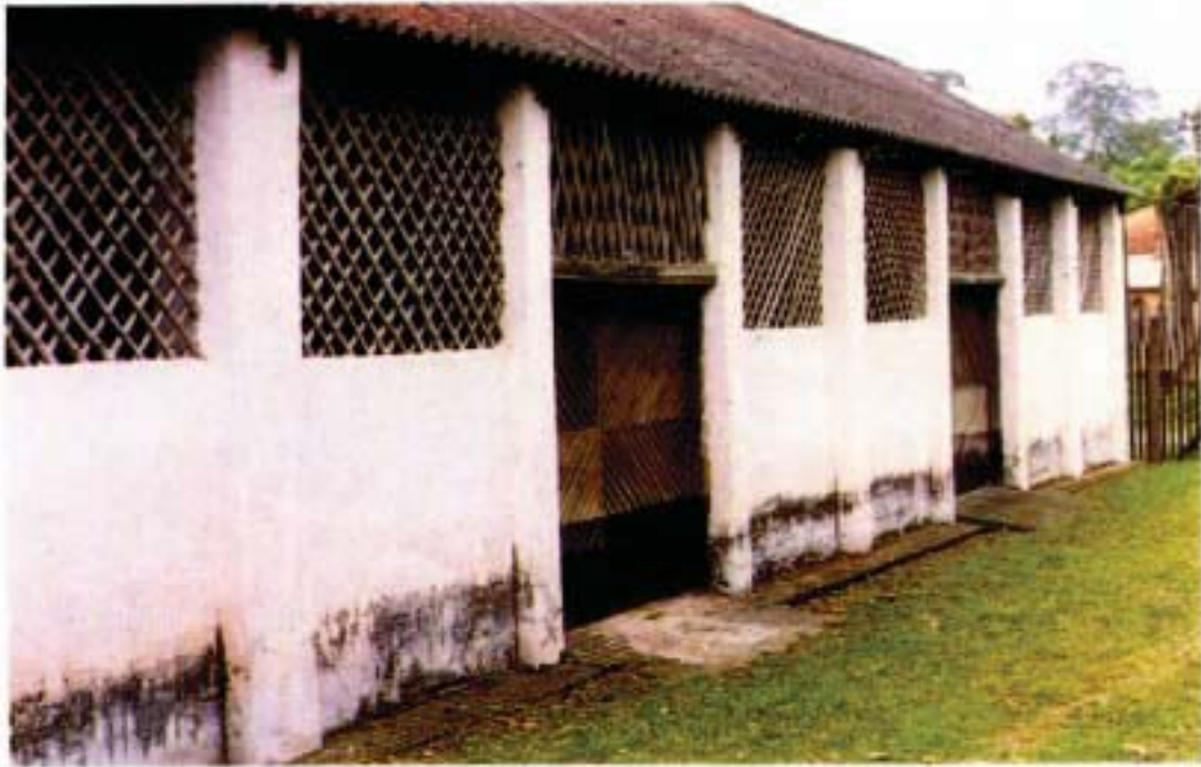
FIGURE 10. Treated bamboos for reinforcing mud walls for storage godowns (erected 1959)
